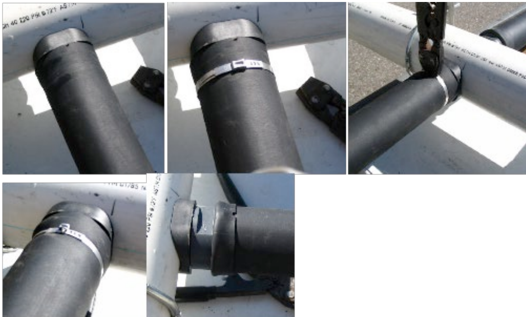
Figure 12: Images of Diffuser Clamp Process
