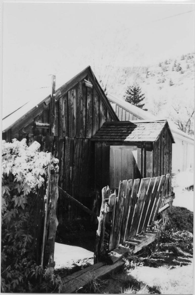
54N. 68.5 Coal Shed/Wood Shed 9/2002
