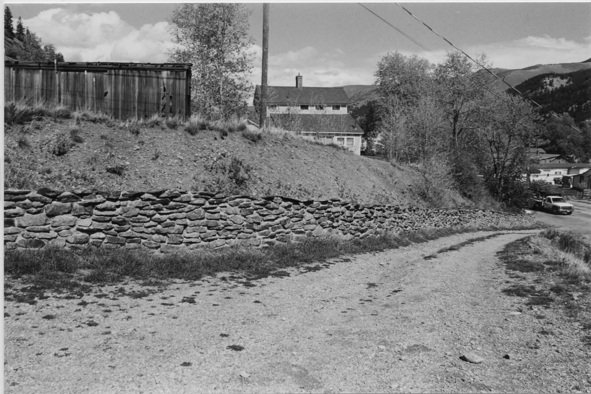
5HN.68.65 stone retaining wall 9/2002
