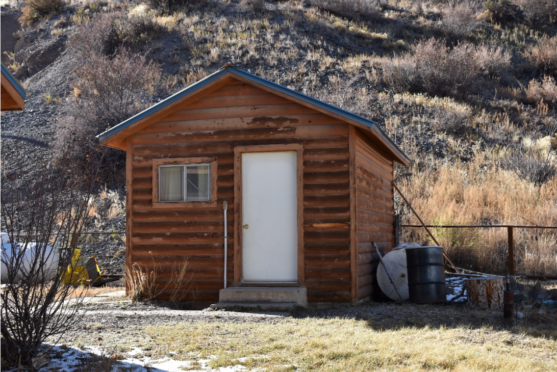
CD 1, Image 27, View to West, of the shed
