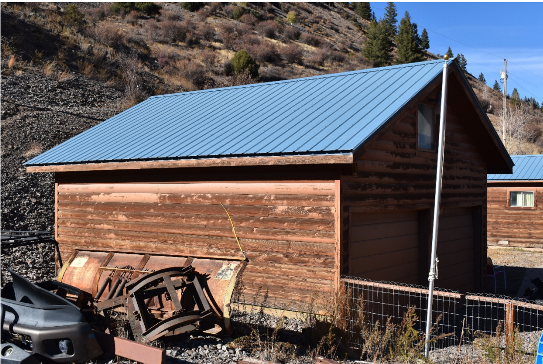
CD 1, Image 28, View to Northwest, of the Garage
