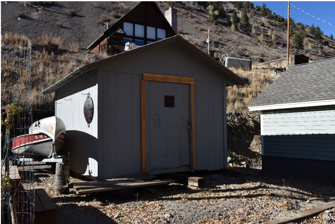
CD 1, Image 22, View to West, of the shed
